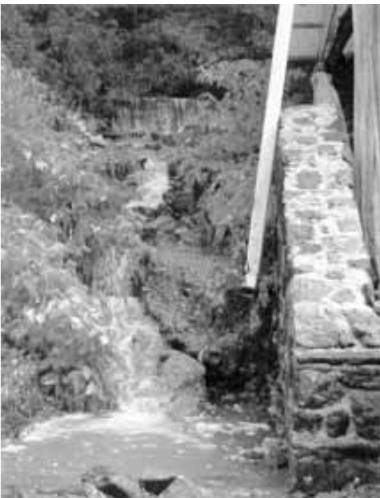
STORMWATER THAT USED TO INUNDATE THE VALLEY GREEN INN (LEFT) IS NOW BEING DIVERTED BY MEASURES SUCH AS THIS HEAD WALL (RIGHT), BUILT BY VOLUNTEERS IN 2007
